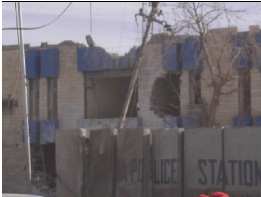
Figure 24 Quriya Police Station after the blast
