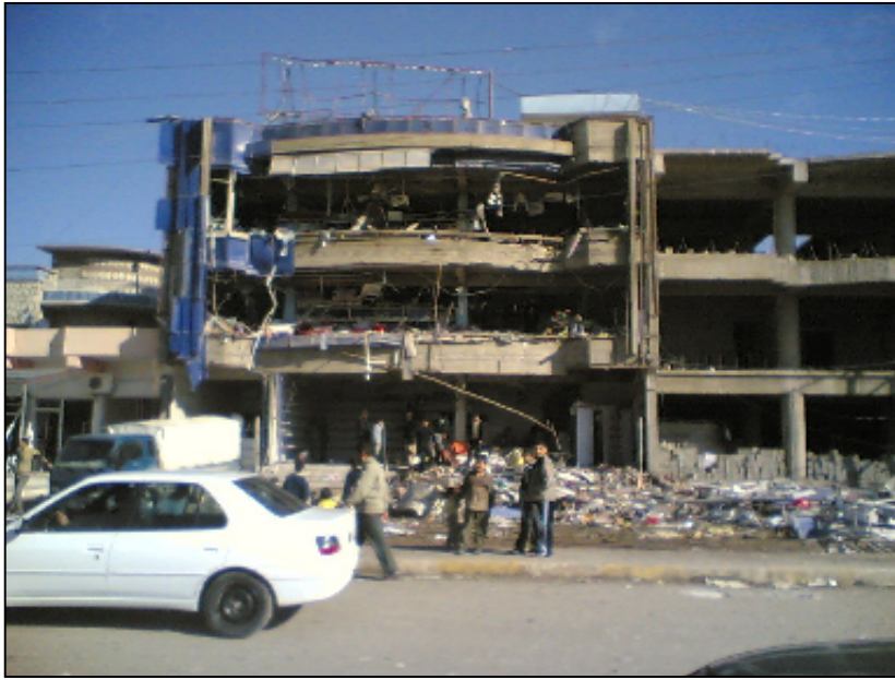
Figure 23. Al_Tasahul supermarket after the explosion
