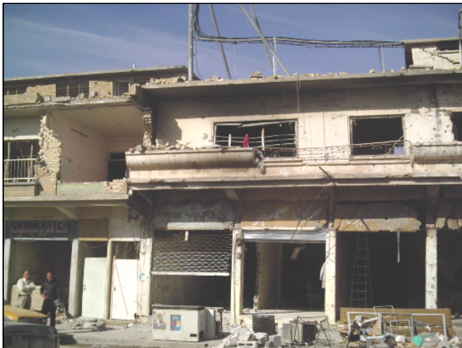
Figure 26. The damage caused by the explosion on Turkmen properties
