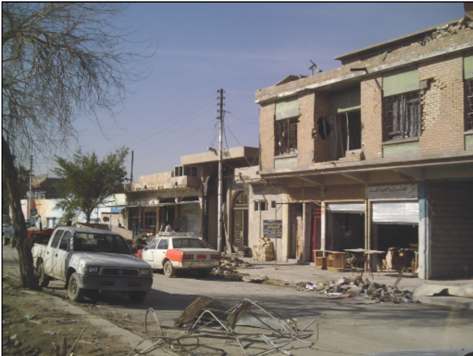
Figure 28. The damaged caused by the explosion on Turkmen properties
