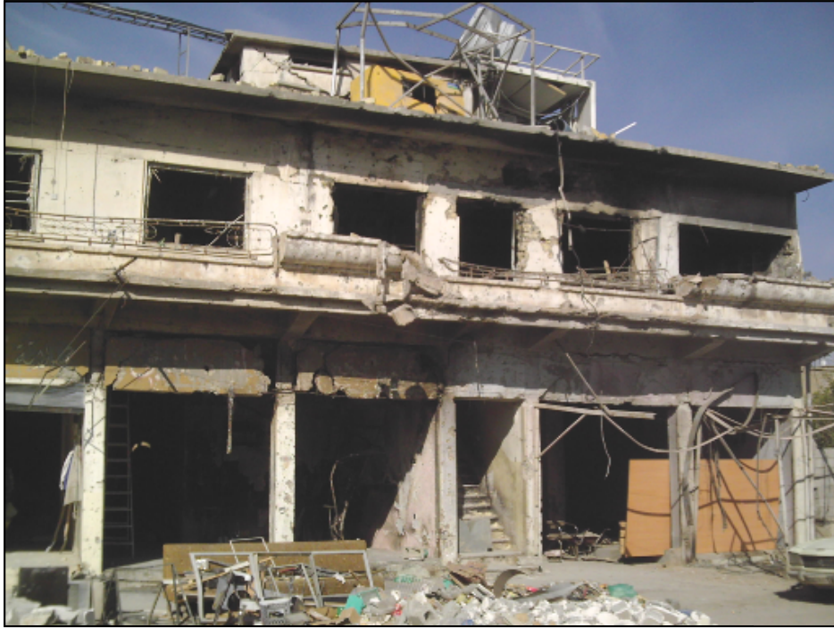
Figure 27. The damage caused by the explosion on Turkmen properties
