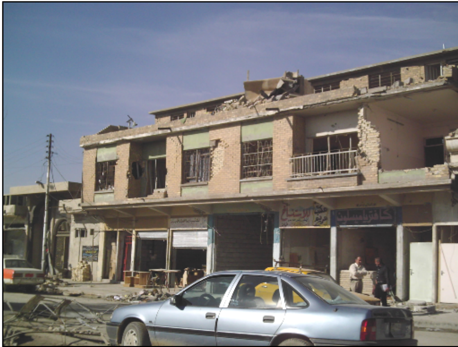
Figure 29. The damage caused by the explosion on Turkmen properties
